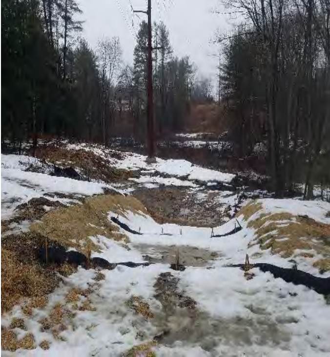
Fig 9: BMPs on access road to Str. 28. Viewing north. (02-27-20).
