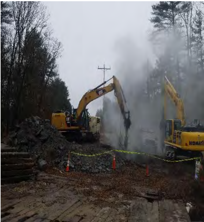
Fig 7: Crew drilling ledge at Str. 66. Viewing west. (02-27-20).
