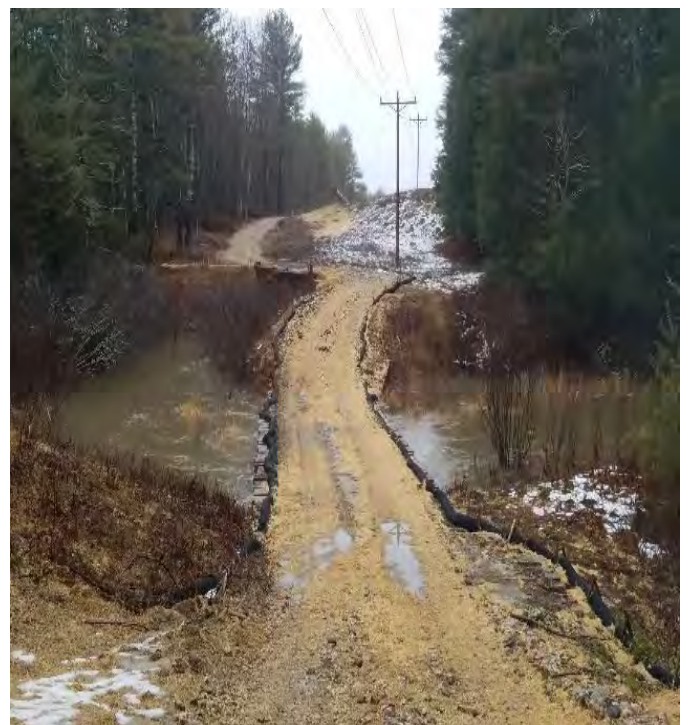
Fig 8: Access road to Str. 52. Over stream DS46. Viewing northeast (02-27-20).
