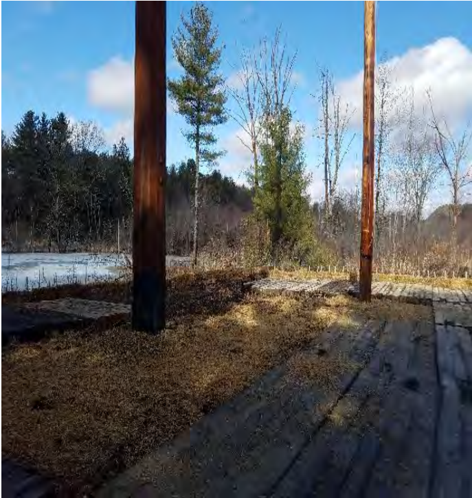
Fig 13: Str. 115 foundation and work area. Viewing north. (02-27-20).
